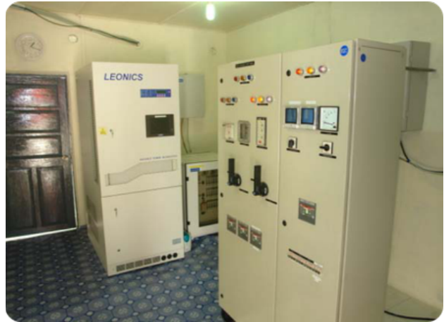
Fig.15 Bidirectional Minigrid Inverter and the Distribution Control panels.
